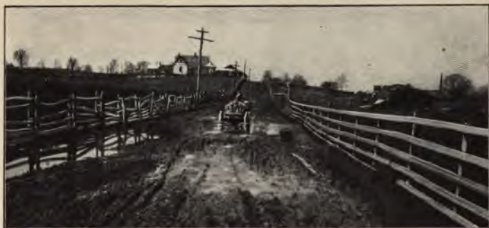
1. The road in its original condition.
